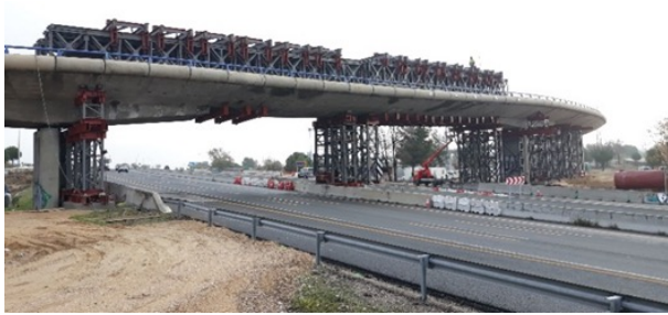
Figure 28. Truss girders for auxiliary structure to dismantle main span over M-40.
