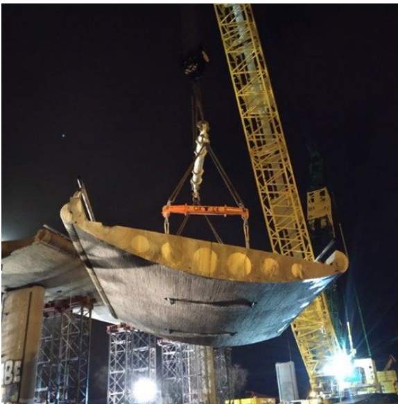
Figure 6. Cross section view of a disassembled segment of typical span.
