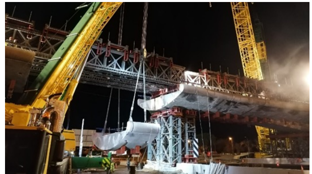
Figure 30. Disassembly of the span over M-40 carriageways.
