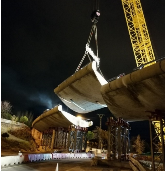
Figure 5. Disassembly of typical span section over M-607 approach ramp.
