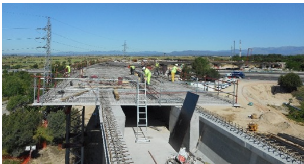
Figure 36. Construction of top slab by means of thin precast slabs over precast U beam.
