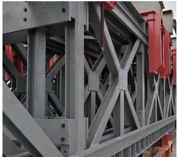
Figure 31. Detail view of truss girders for auxiliary structure.
