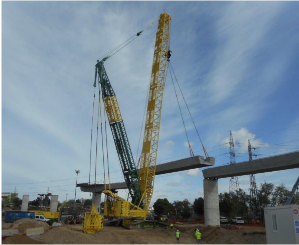
Figure 34. Crawler crane during beams placement.
