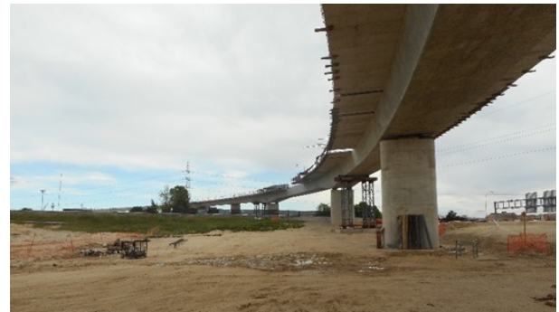
Figure 46. Bottom view of the new deck during construction.
