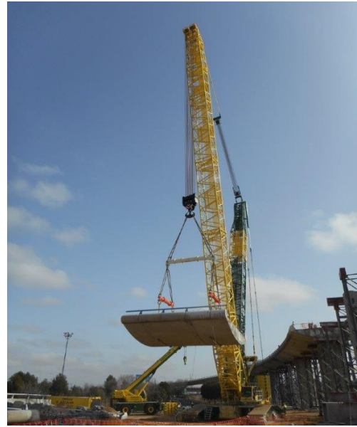
Figure 29. High-capacity crawler crane during disassembly operations.
