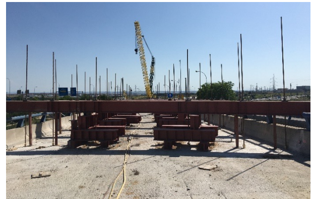
Figure 26. Auxiliary steel structure to tie deck cross section over railway lines.
