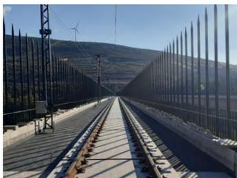
FOTO DE PORTADA: Aerial view of the Tuela Viaduct (Pedralba-Campobeceros section of the Madrid-Galicia HS line, Spain). Precast slabs of VP-AFTRAV ballastless track system. Courtesy by PRECON and Ferrovial.
