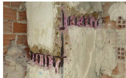
Figure 7. Example of a column where the carbonate concrete has reached the position of the rebars.
