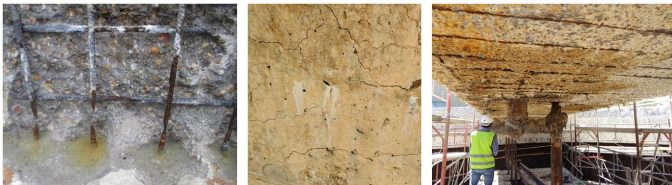
**Figure 8.** Different causes of deterioration of reinforced concrete: pitting corrosion (left), AAR (centre), acid attacks (right).
