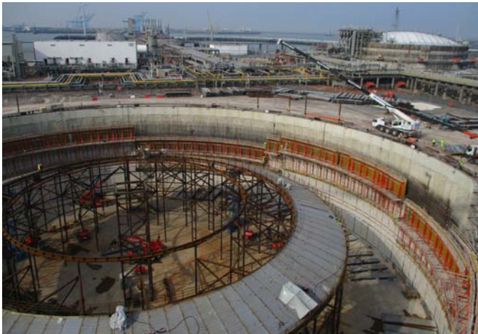
Vista general muro exterior
