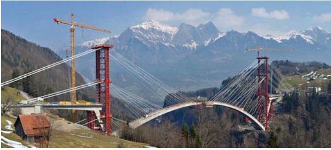
Figure 1. Tamina Canyon Bridge, Switzerland
