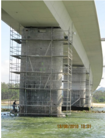
Cathodic protection wiring installation of a pile
