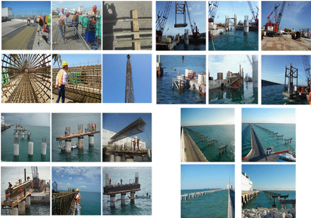
Figure 8. Construction process photographs: substructure construction stage.
