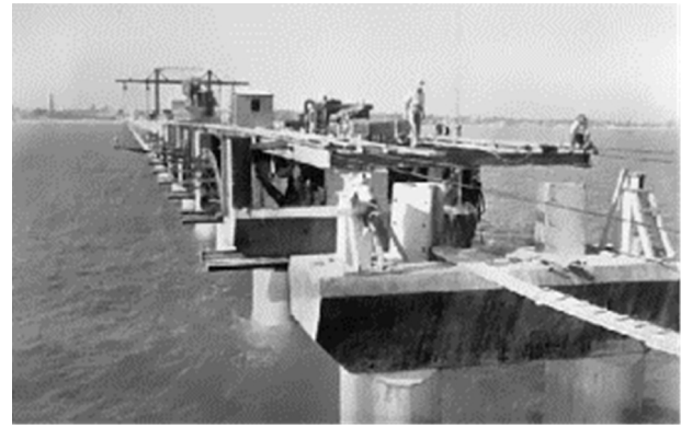
Figure 1. View of cross girders and piles during the construction process.
