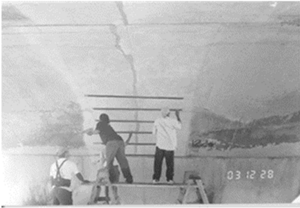
Figure 4. Rehabilitation of one of the cracked arches.
