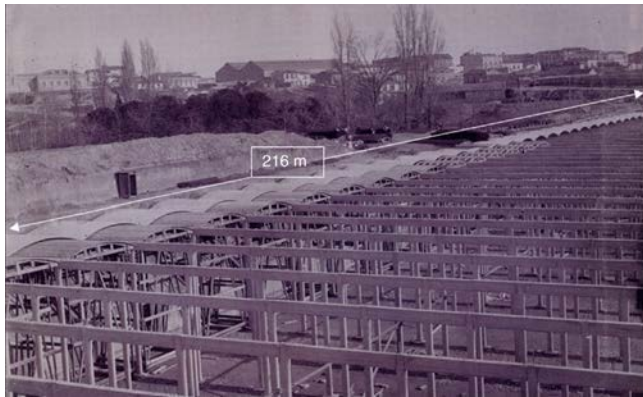
Figure 6. Construction of the Third Reservoir of Canal de Isabel II. Madrid, 1905.
