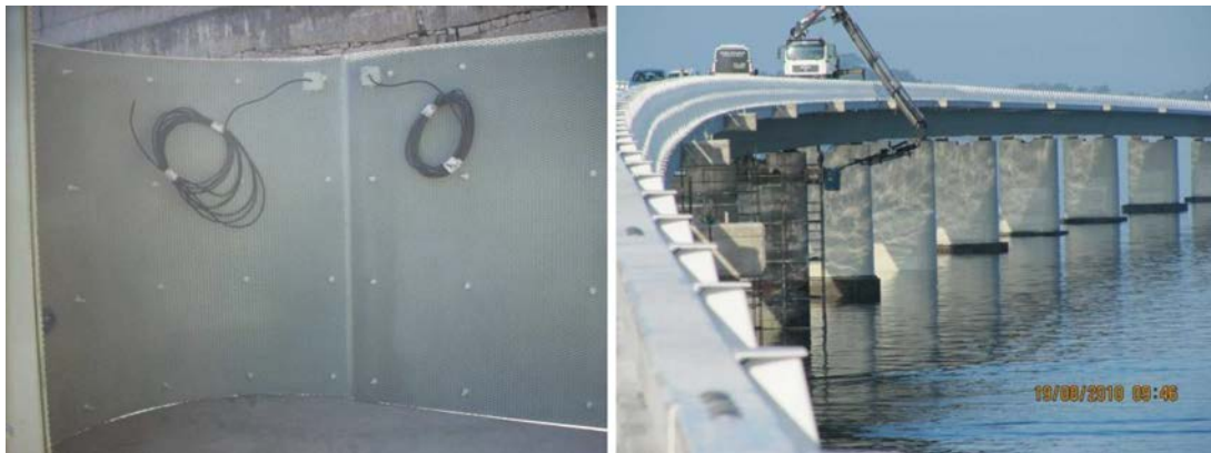
Figure 7. Repair of the piles with the Fosroc jackets.
