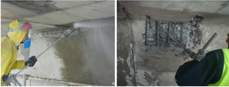
Figure 4. Techniques of demolition of damaged areas of the deck.
