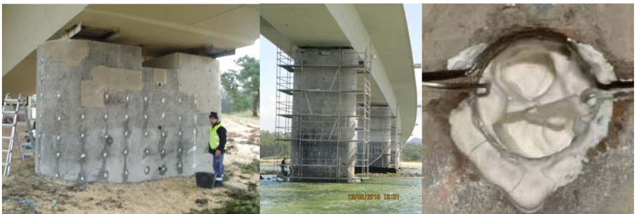
Figure 8. Repair of the piles with conventional technique and CPT cathodic protection.
