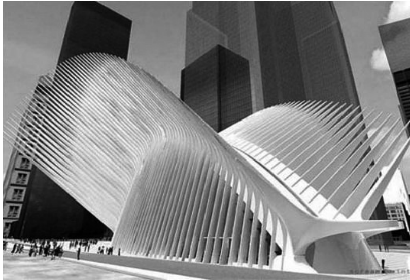
Santiago Calatrava. Path Station , New York.
