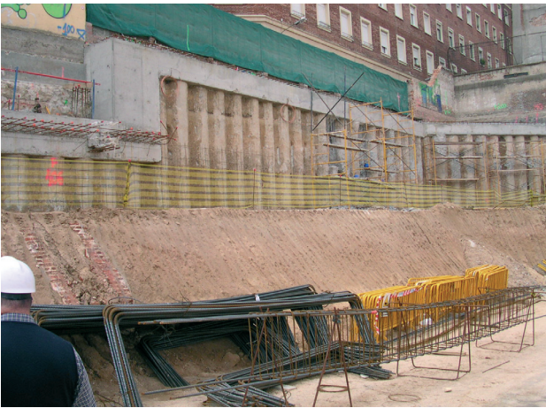
Figura 31. Contención perimetral del solar. Figure 31. Retaining wall.
