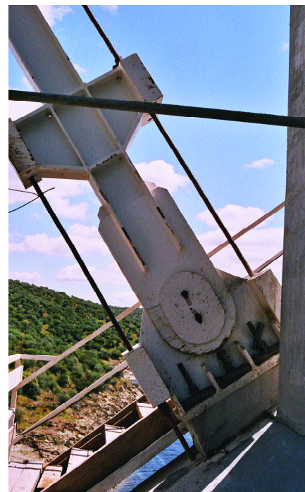
Fig.42. Detalle de tesado de diagonal rígida. Fig.42. Detail of rigid diagonal tensioning.
