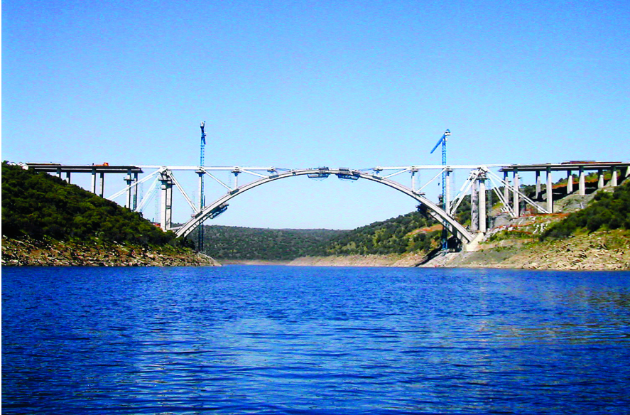
Fig.32. Apertura en clave. Fig.32. Crown opening.
