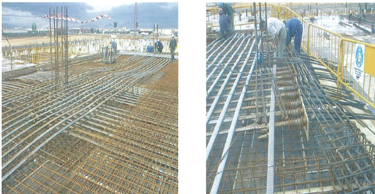
Figura 17. Vista general pretensado de planta primera. Figure 17. General view of prestressed slab.
