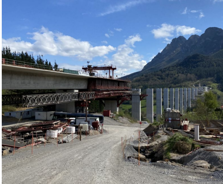
Figure 1. Construction of a bridge with an underslung MSS.
