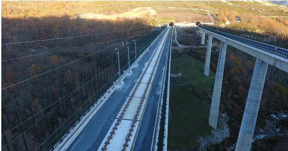
Figure 1. Aerial view of the Tuela Viaduct (Pedralba-Campobecerros section of the Madrid-Galicia HS line, Spain). Precast slabs of VP-AFTRAV ballastless track system. Courtesy by PRECON and Ferrovial.
