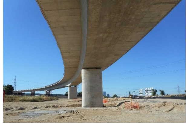
Figure 48. View of the bridge after completion
