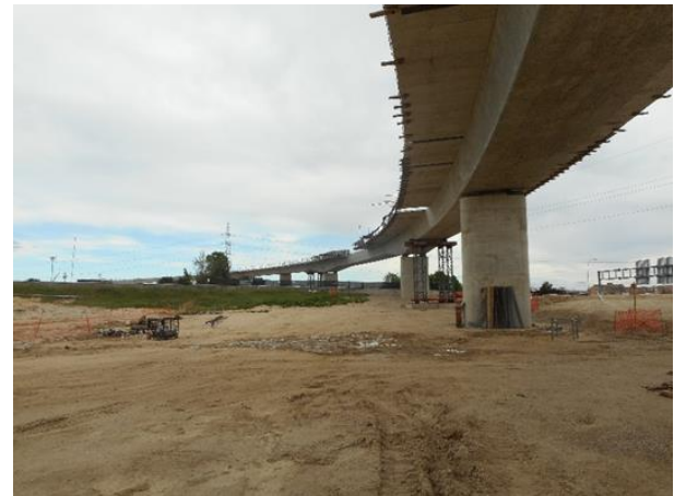
Figure 46. Bottom view of the new deck during construction
