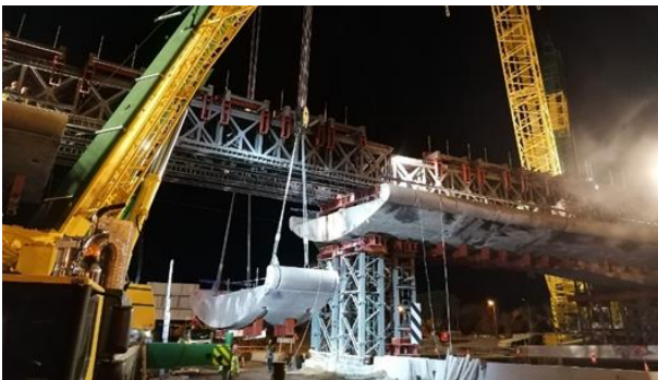
Figure 30. Disassembly of the span over M-40 carriageways
