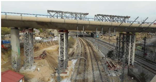
Figure 23. Phase 17: Disassembly of span 16 over railway line
