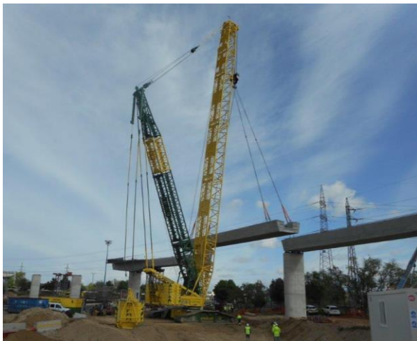
Figure 34. Crawler crane during beams placement
