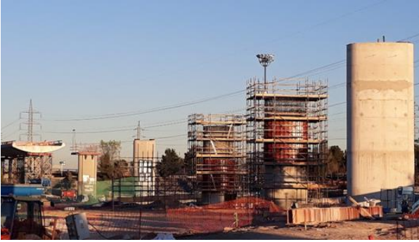
Figure 47. Rehabilitation of piers before deck construction
