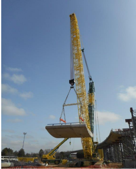
Figure 29. High-capacity crawler crane during disassembly operations
