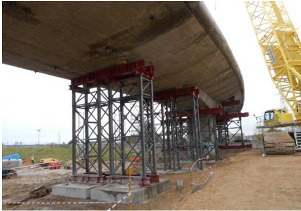
Figure 4. Temporary steel towers to support existing deck sections.
