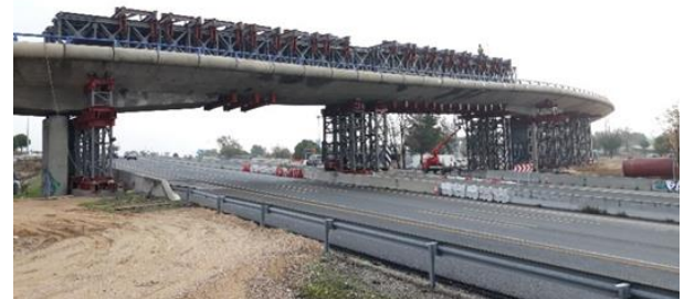
Figure 28. Truss girders for auxiliary structure to dismantle main span over M-40
