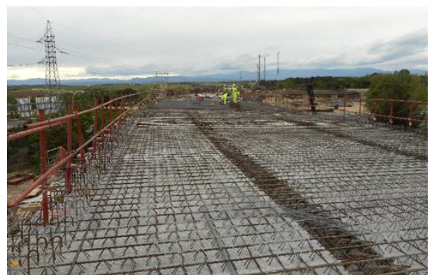
Figure 38. Top slab during reinforcing installation
