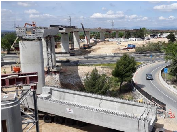
Figure 32. Precast beam before installation
