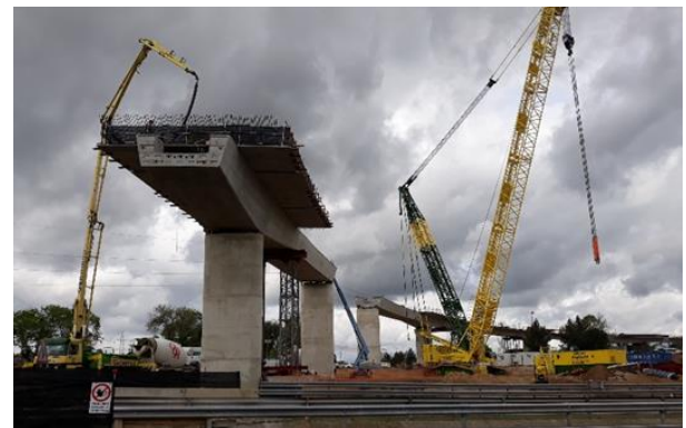
Figure 33. Construction of new deck over M-607 carriageways
