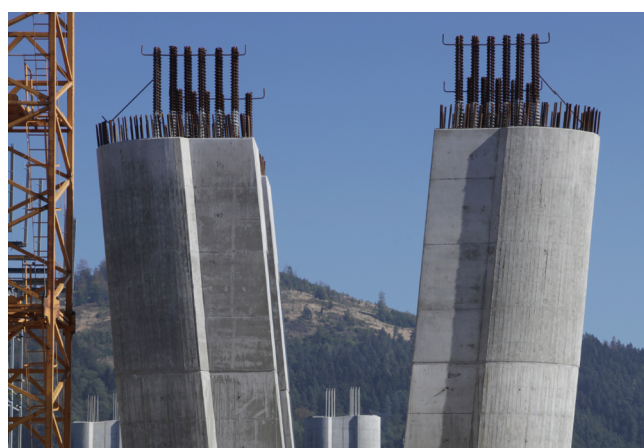
Figure 17. Piers of the Bridge across the River Vah's Reservoir.
