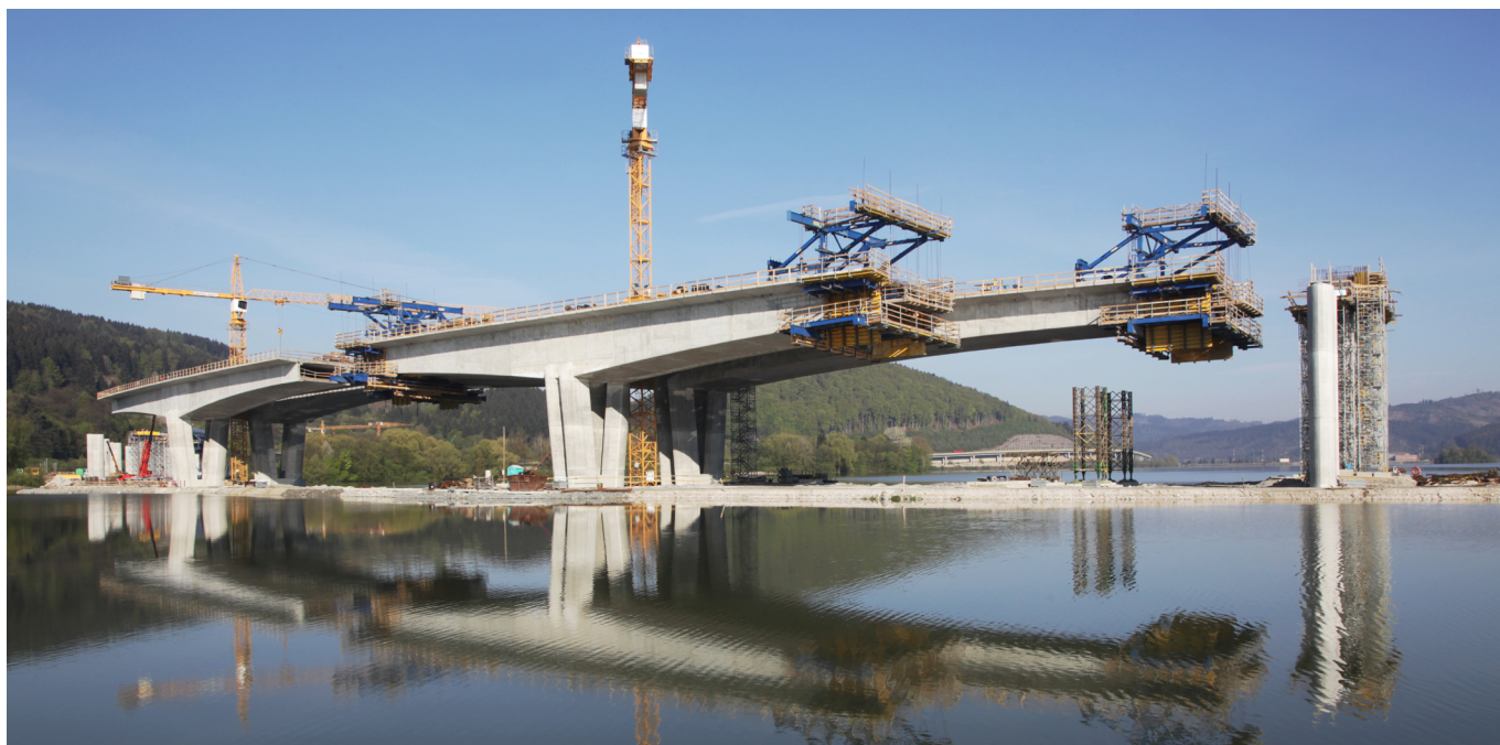
Figure 14. Cantilever construction of the Bridge across the River Vah's Reservoir.
