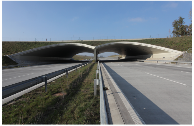
Figure 27. Wildlife Overpasses, Czech Republic.
