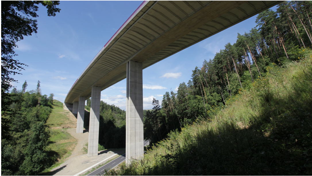
Figure 2. Bridge across the Lodina Creek Valley.
