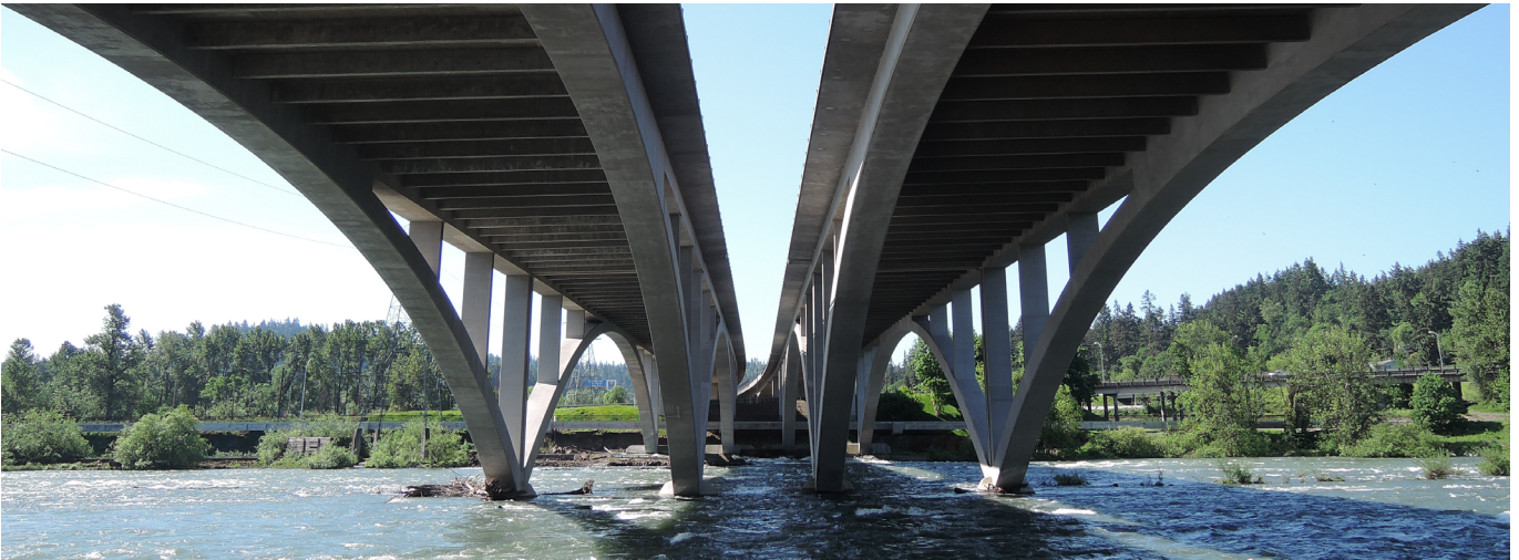
Figure 30. Willamette River Bridge.
