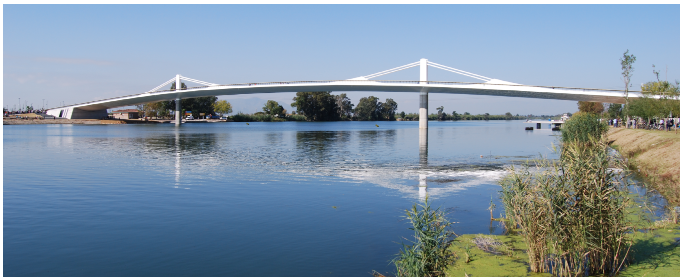
Figure 23. Bridge across the River Ebro.
