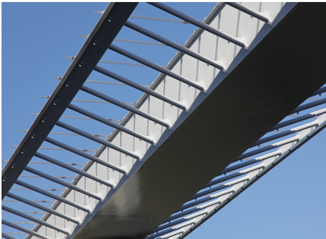
Figure 8. Steel structure - Bridge across the Kremlice Creek Valley.
