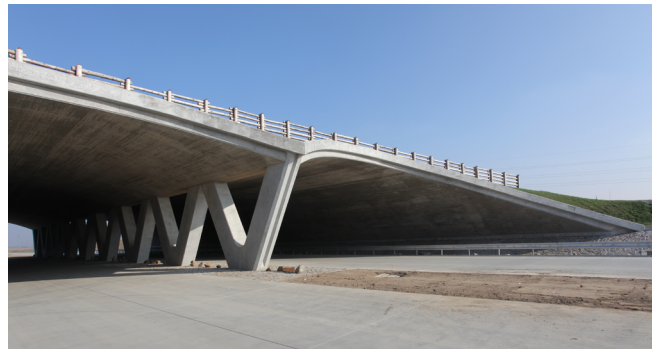
Figure 28. Wildlife Overpasses, Czech Republic.
