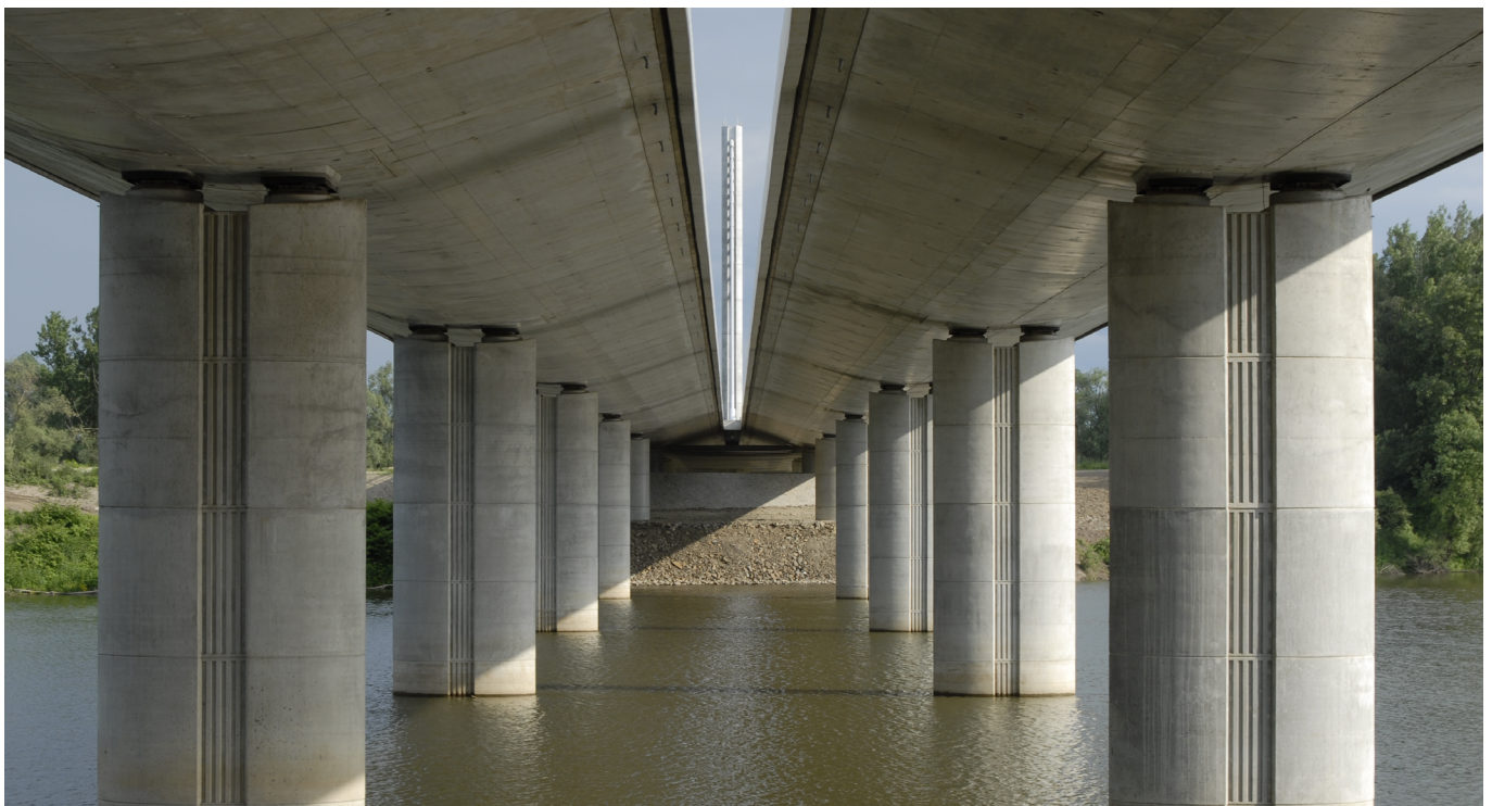
Figure 19. Deck of the viaducts - Bridge across the Odra River.
