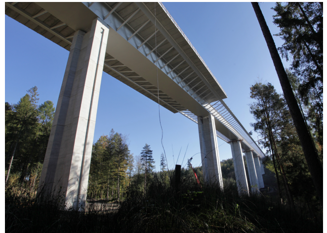
Figure 9. Progressive erection of the deck - Bridge across the Kremlice Creek Valley.
