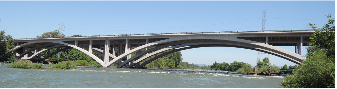
Figure 29. Willamette River Bridge.
