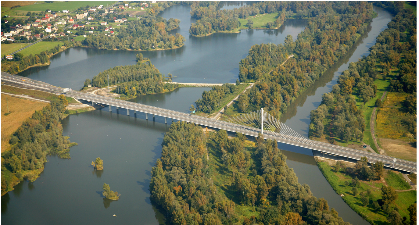
Figure 18. Bridge across the Odra River.
