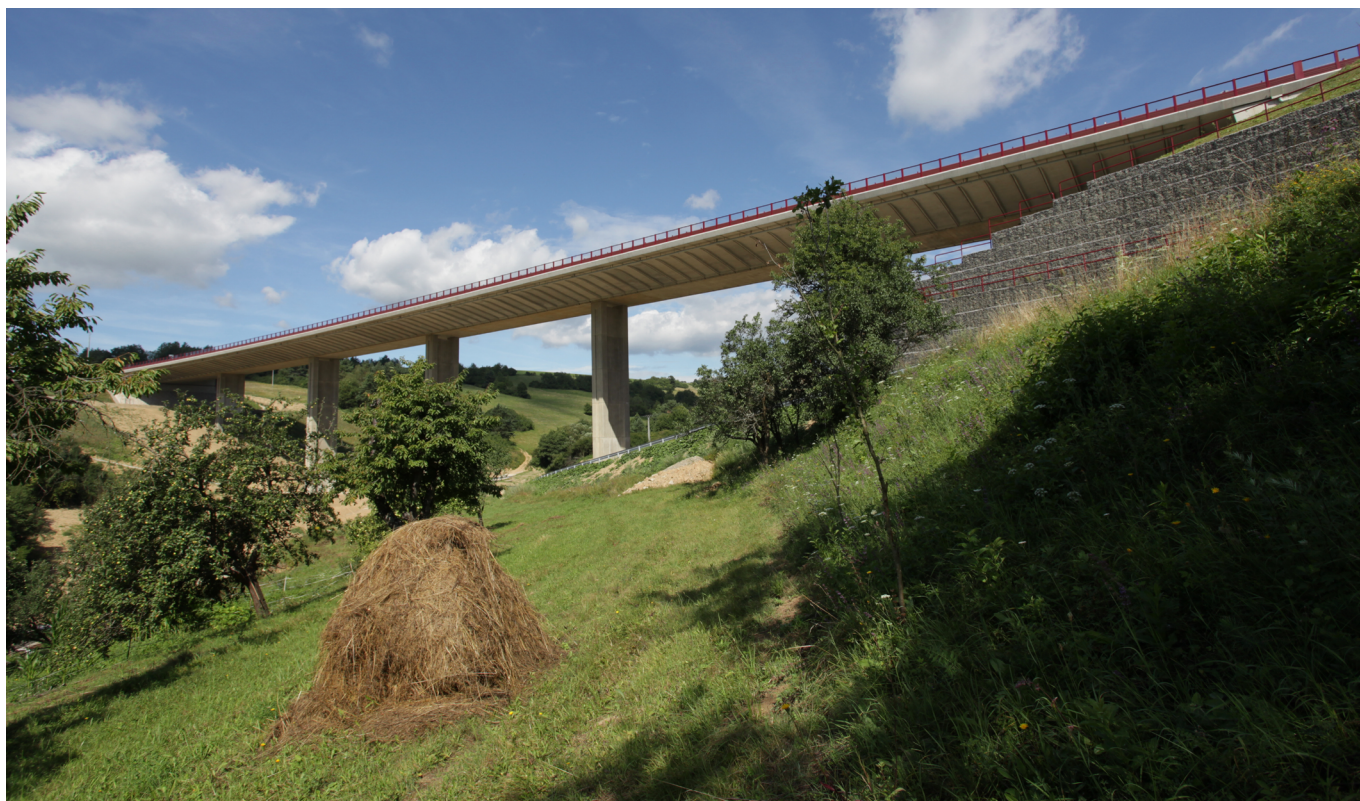
Figure 1. Bridge across the Lazny Creek Valley.
