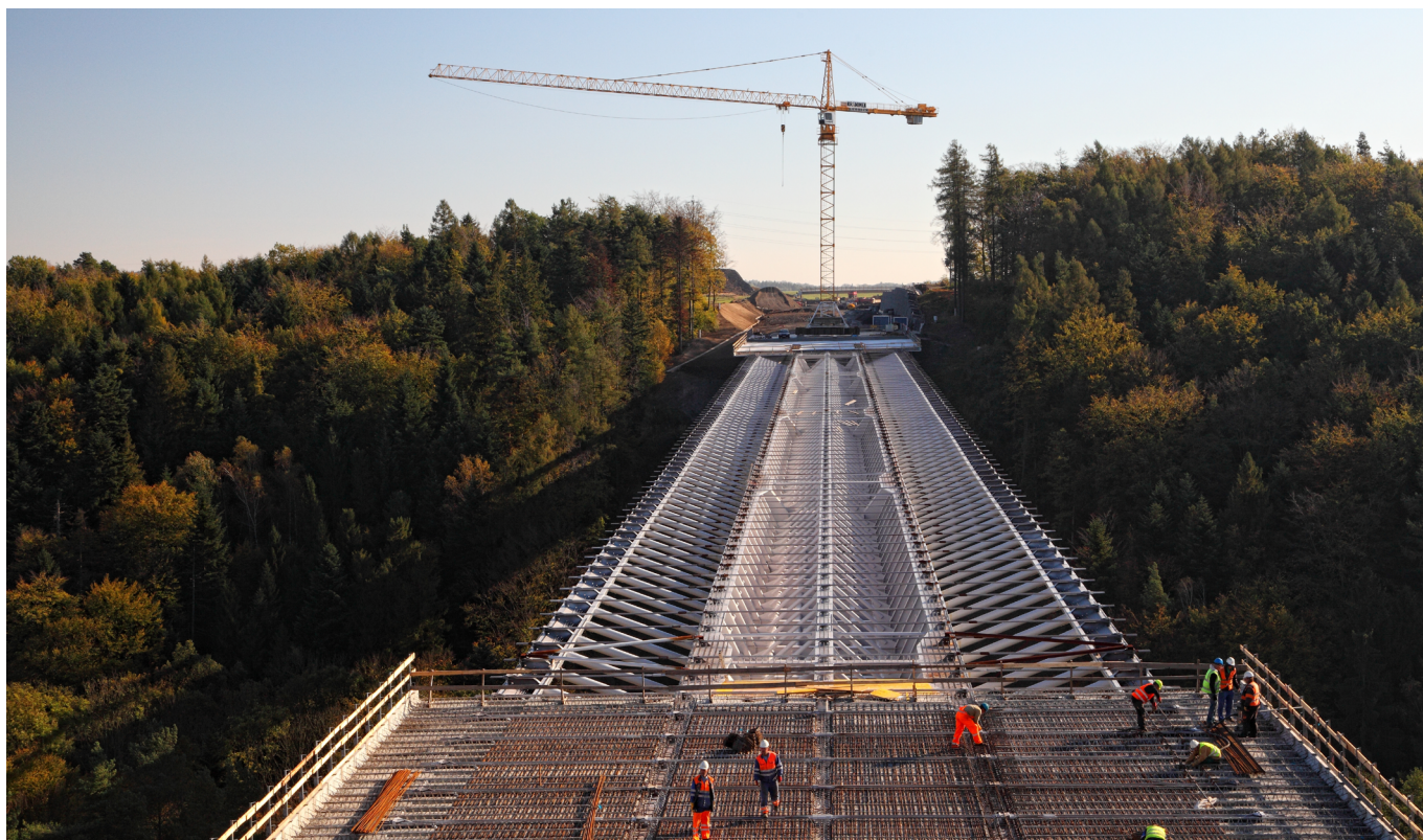
Figure 10. Progressive casting of the deck - Bridge across the Kremlice Creek Valley.
