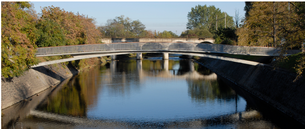
Figure 35. Svatka River Pedestrian Bridge.
