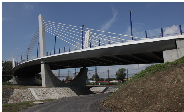
Figure 21. Bridge across the Railway Station at Bohumin.
