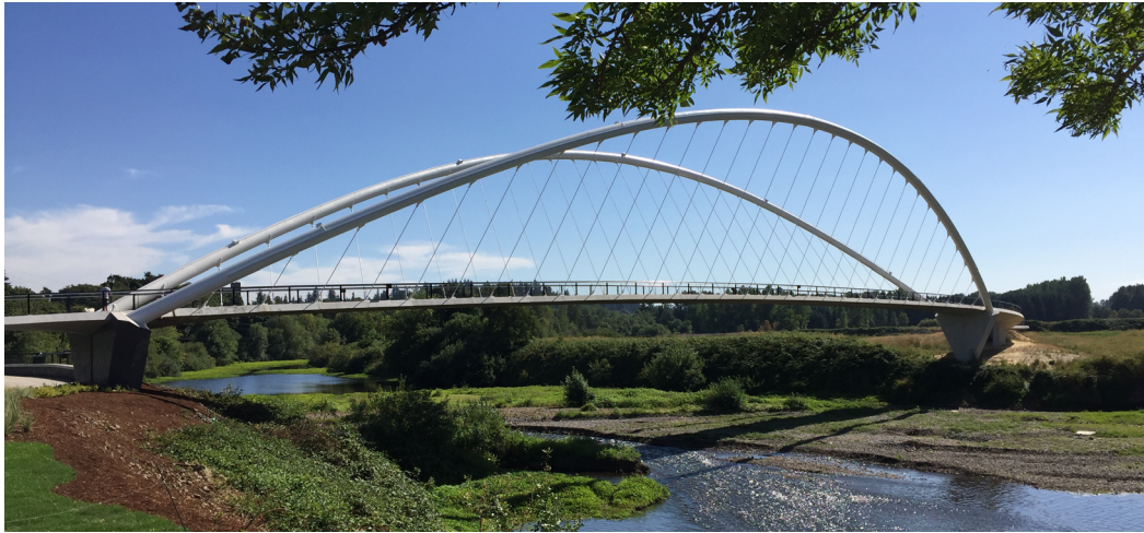
Figure 34. Minto Island Pedestrian Bridge.
