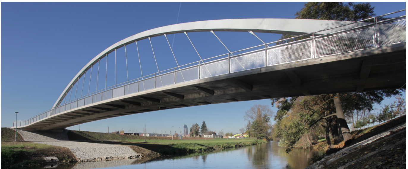
Figure 33. Brno-Komarov Pedestrian Bridge.
