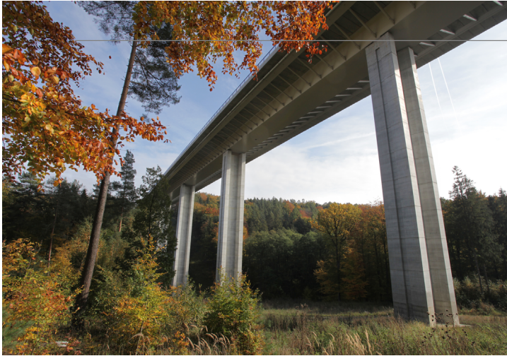
Figure 6. Bridge across the Kremlice Creek Valley.
