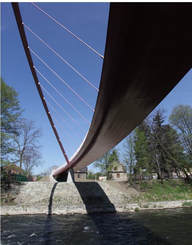
Figure 31. Pedestrian Bridge across the Olse River.
