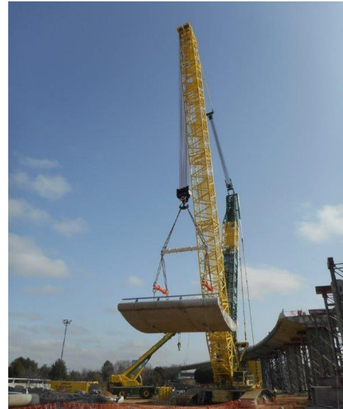
Figure 29. High-capacity crawler crane during disassembly operations.
