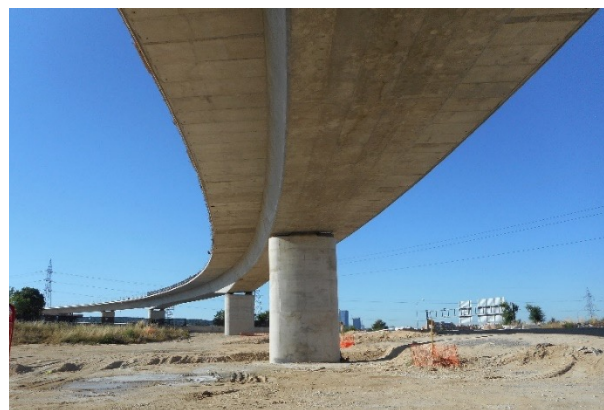
Figure 48. View of the bridge after completion.
