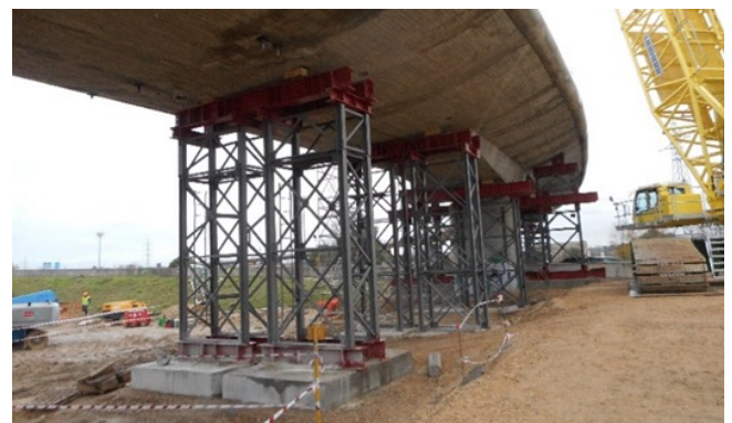
Figure 4. Temporary steel towers to support existing deck sections.
