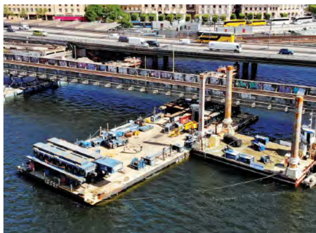
Figure 1. Detail of removal old section in Stockholm.
