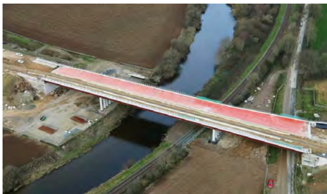
Figure 2. Completed structure with finishing works on-going.
