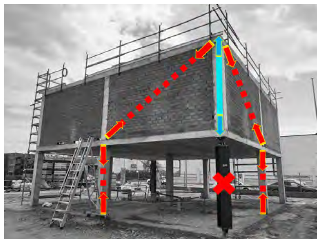
Figure 2. Activation of an alternative load path based on the infill masonry walls.
