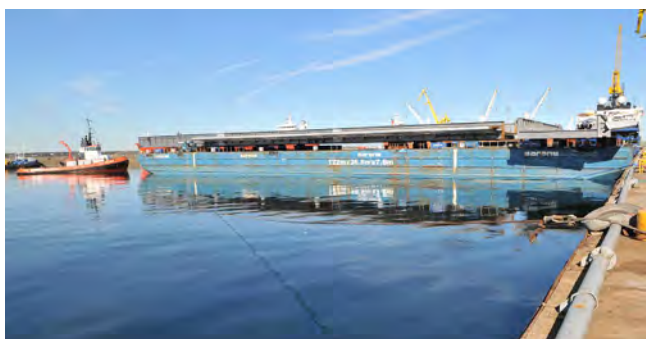
Figure 2. Load outs of three new bridge sections at Tallinn by means of SPMTs on Caroline SARENS 400ft barge.
