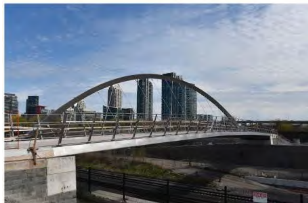
Figure 2. View of North Bridge looking South.
