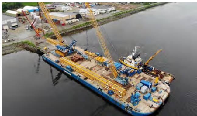
Figure 2. Assembly of CC8800 on SARENS barge.
