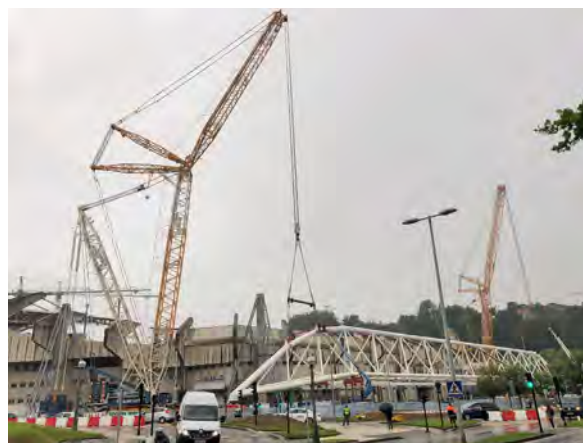
Figure 1. Initial position of the cranes for taking the load.
