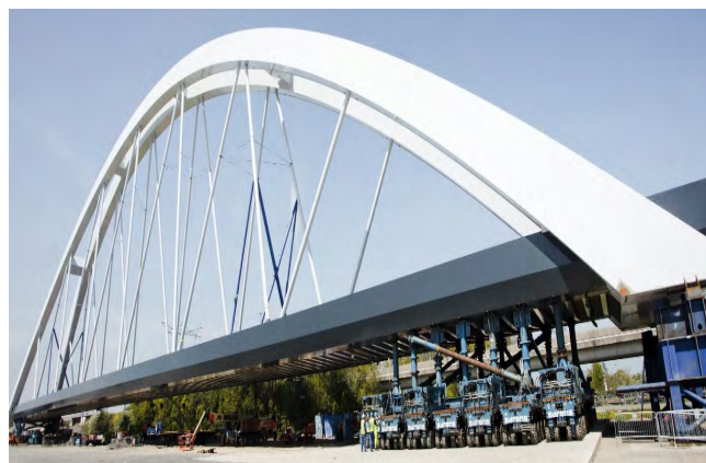
Figure 1. SPMT arrangement on north side.
