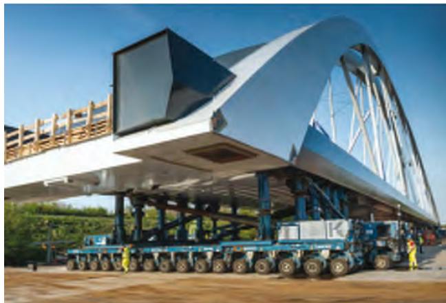
Figure 2. SPMT arrangement on south side.
