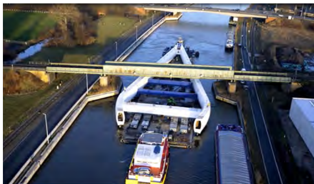
Figure 1. Pylon passing under canal bridge.
