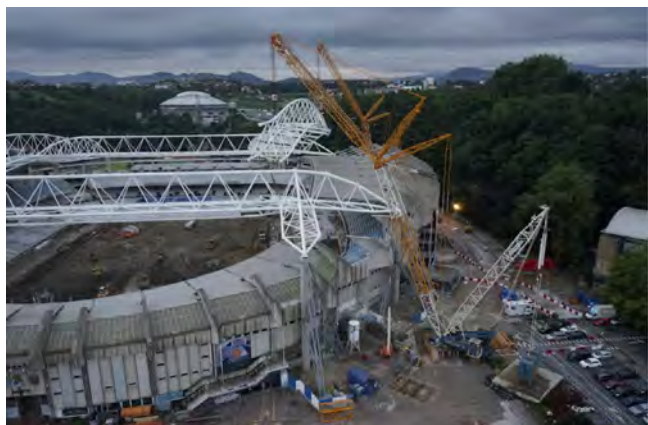
Figure 2. Intermediate position with hooks of both cranes already inside the stadium.
