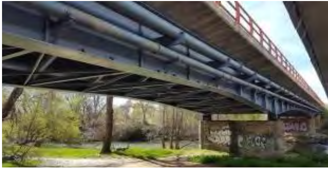
Figure 1. General view, Jarama Bridge.
