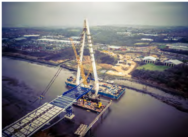
Figure 2. Pylon right after ending the tilting.
