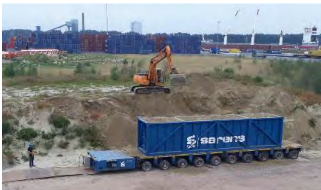
Figure 2. Filling of counterweight.
