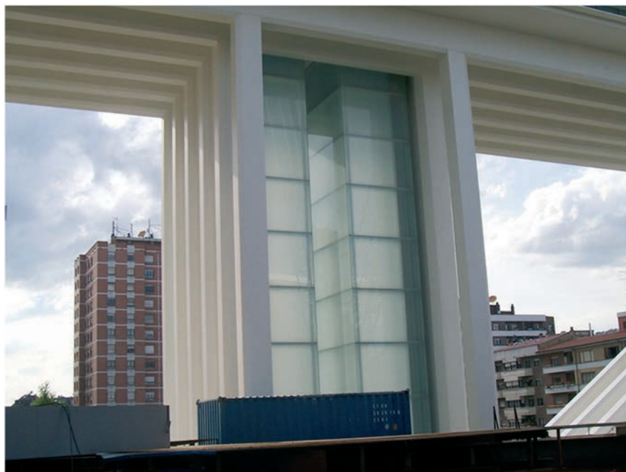
Figura 5. Núcleos acristalados de comunicación vertical Figure 5. Glass-covered cores of vertical circulation
