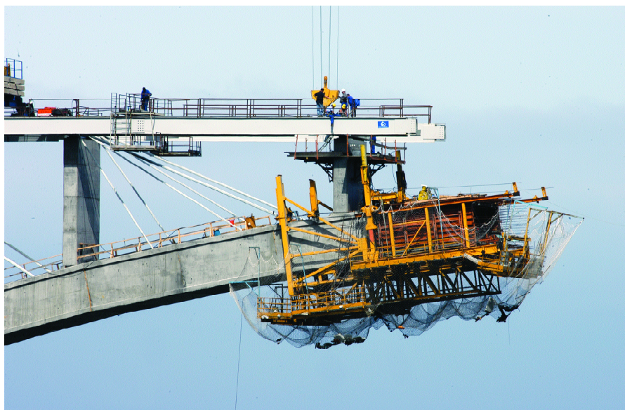
Figura 11. Diagonales auxiliares. Figure 11. Auxiliary diagonals.
