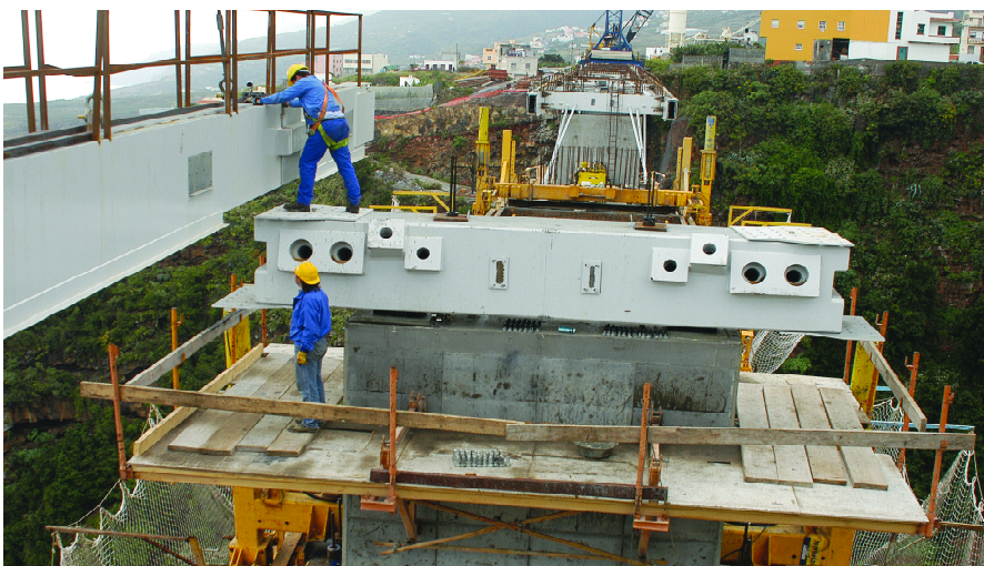
Figura 15. Riostra de pila. Figure 15. Column bracing.
