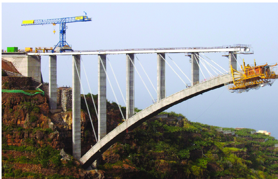
Figura 10. Avance en voladizo con diagonales temporales. Figure 10. Progress in cantilever with temporary diagonals.
