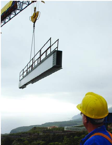
Figura 14. Montaje viga longitudinal. Figure 14. Longitudinal beam assembly.
