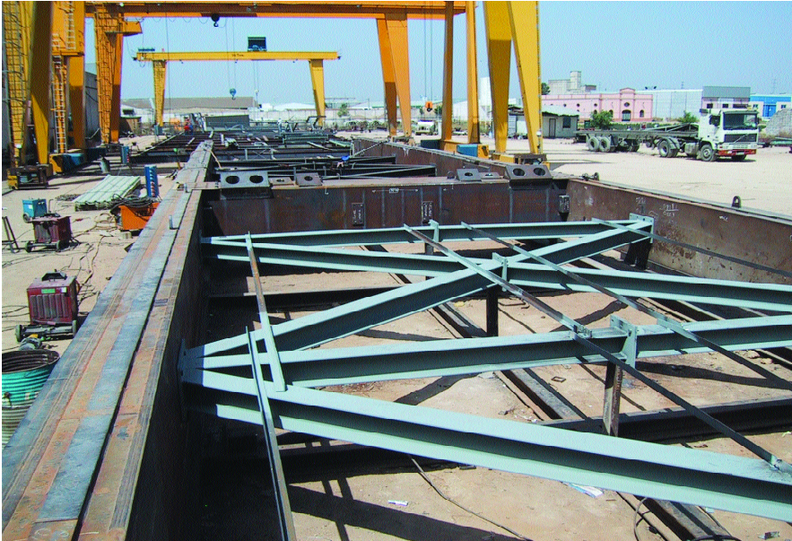
Figura 16. Arriostramiento horizontal. Figure 16. Cross bracing.
