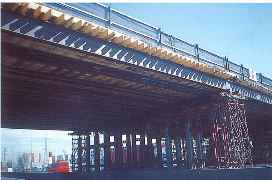
Figura 11. Autocimbra sobre la N-IV. Figure 11. Travelling shutter over the N-IV.
