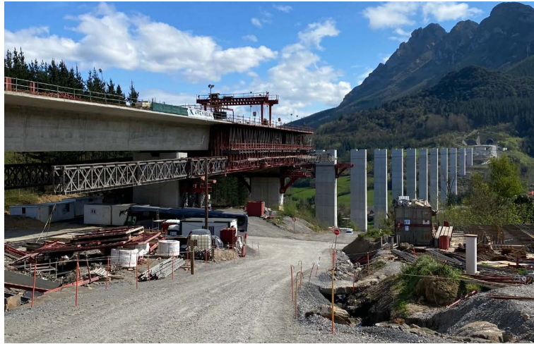
Figure 1. Construction of a bridge with an underslung MSS.
