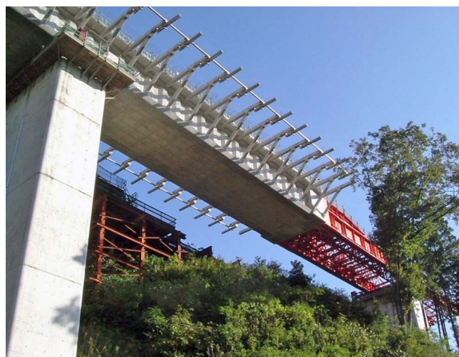
Figure 11. Katsurajima Viaduct by incremental launching of core segments.
