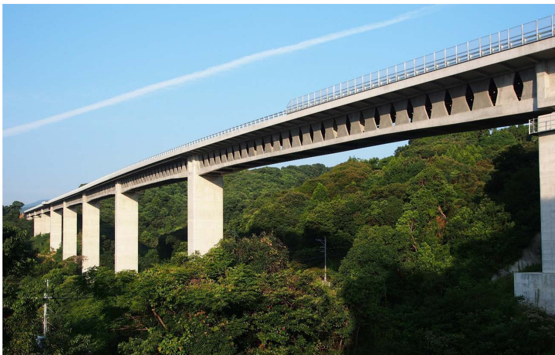
Figure 16. Takubogawa Bridge with butterfly web.
