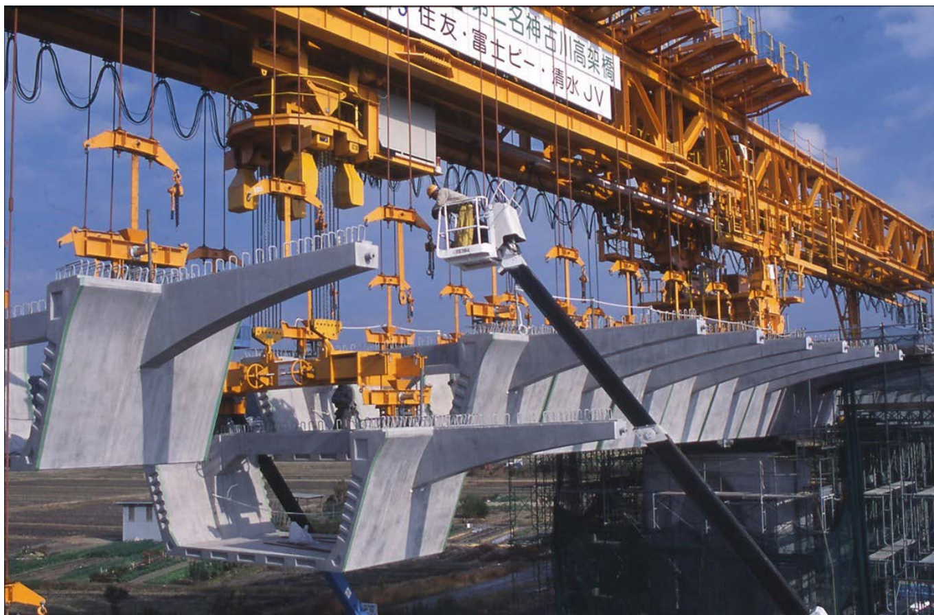
Figure 10. Erection of U-shaped core segments.
