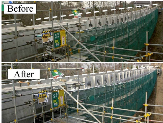
Figure 21. Adjustment of girder alignment using secondary cables.
