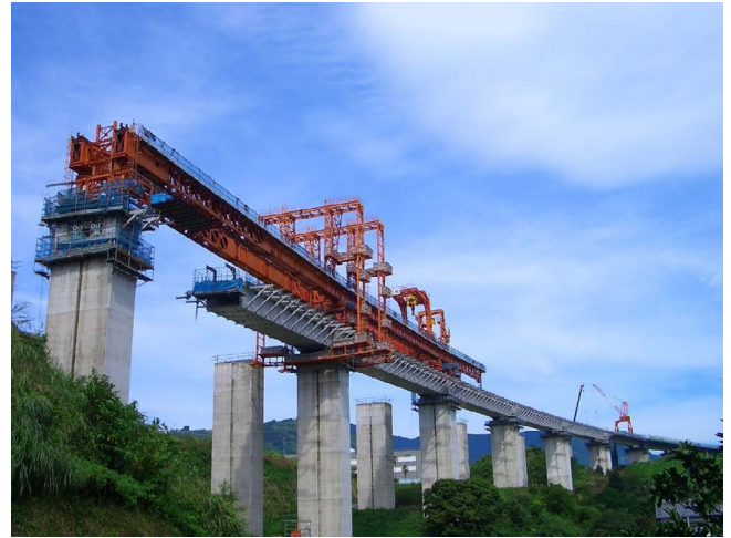
Figure 18. Precast segment cantilevering with erection girder.
