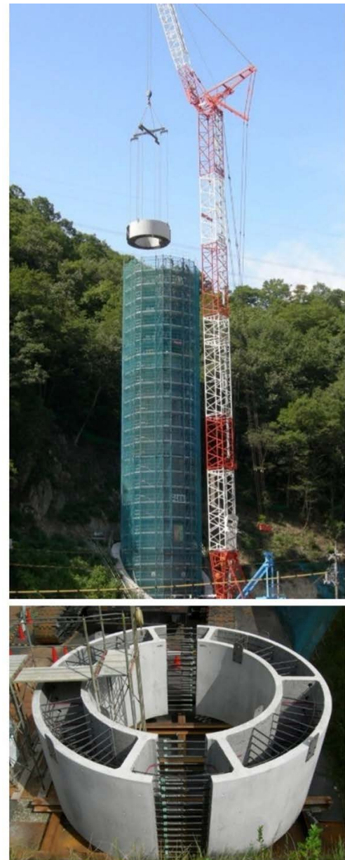
Figure 23. Half precast erection of 80m high pier.
