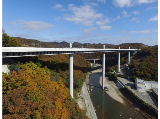
Figure 22. Mukogawa Bridge with lightweight structure.
