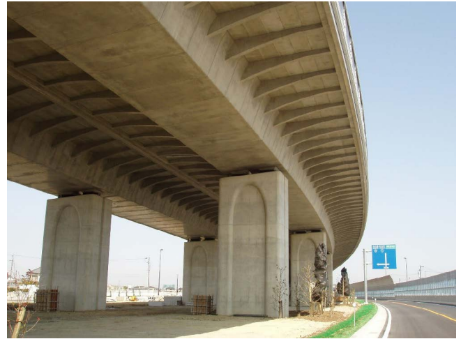
Figure 9. Furukawa Viaduct with factory fabricated segments.
