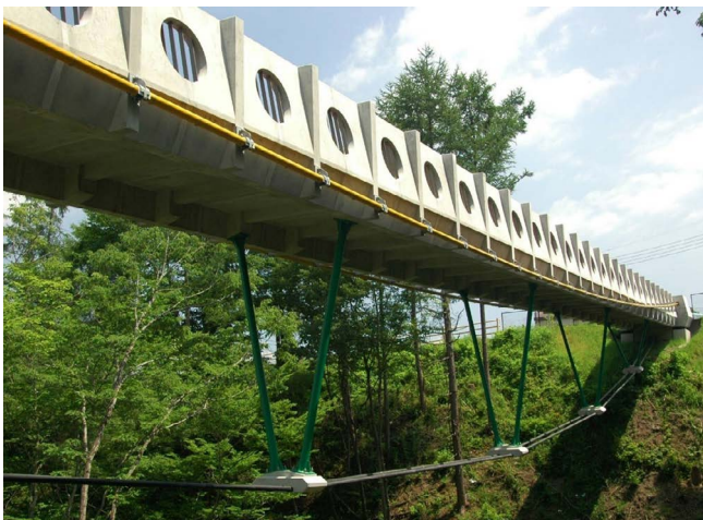
Figure 19. Seishun Bridge with double suspension cables.
