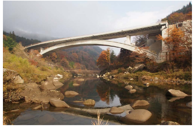
Figure 13. Kakehashi Ichigou Bridge with concrete arch.
