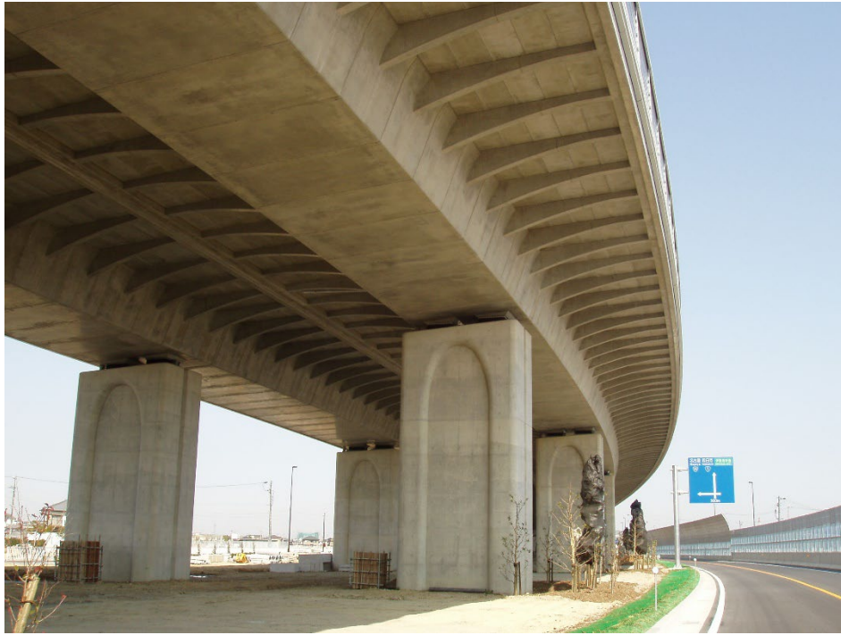
Figure 9 Furukawa Viaduct with factory fabricated segments
