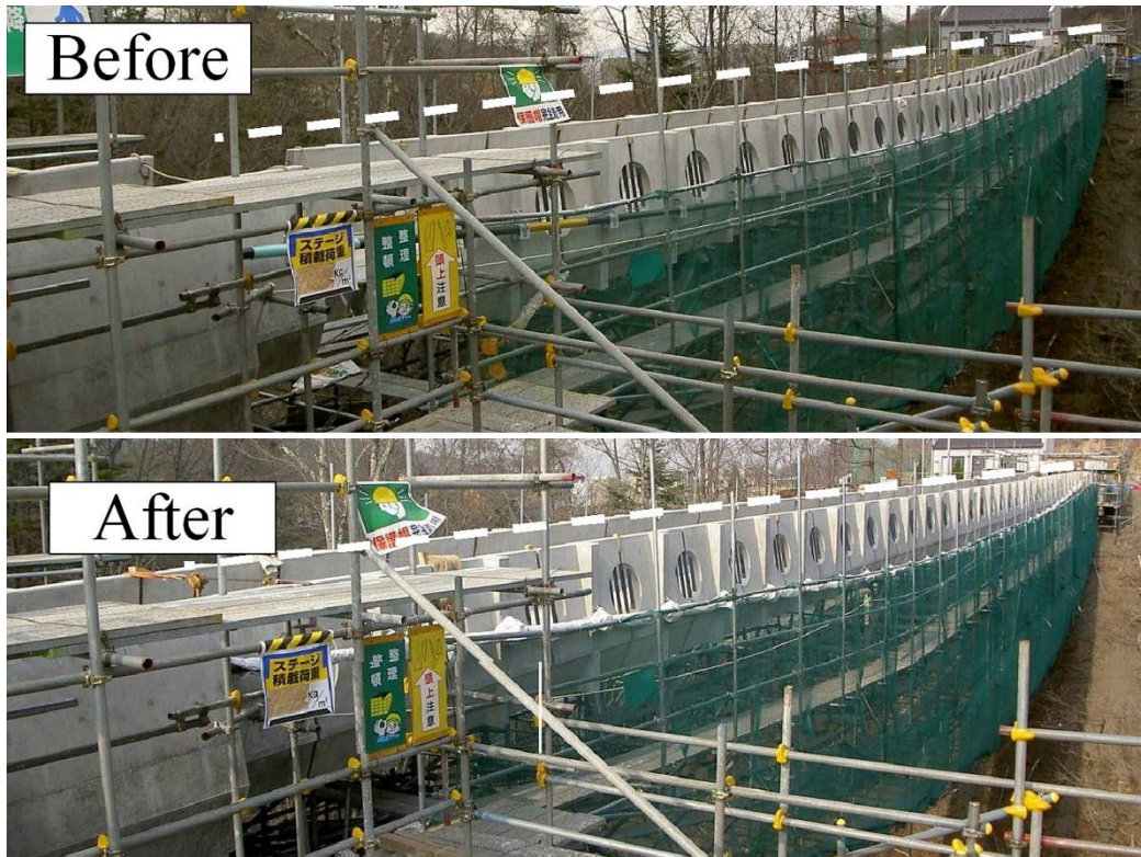
Figure 21 Adjustment of girder alignment using secondary cables
