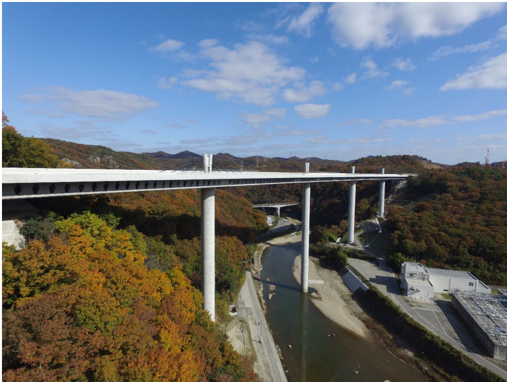
Figure 22 Mukogawa Bridge with lightweight structure
