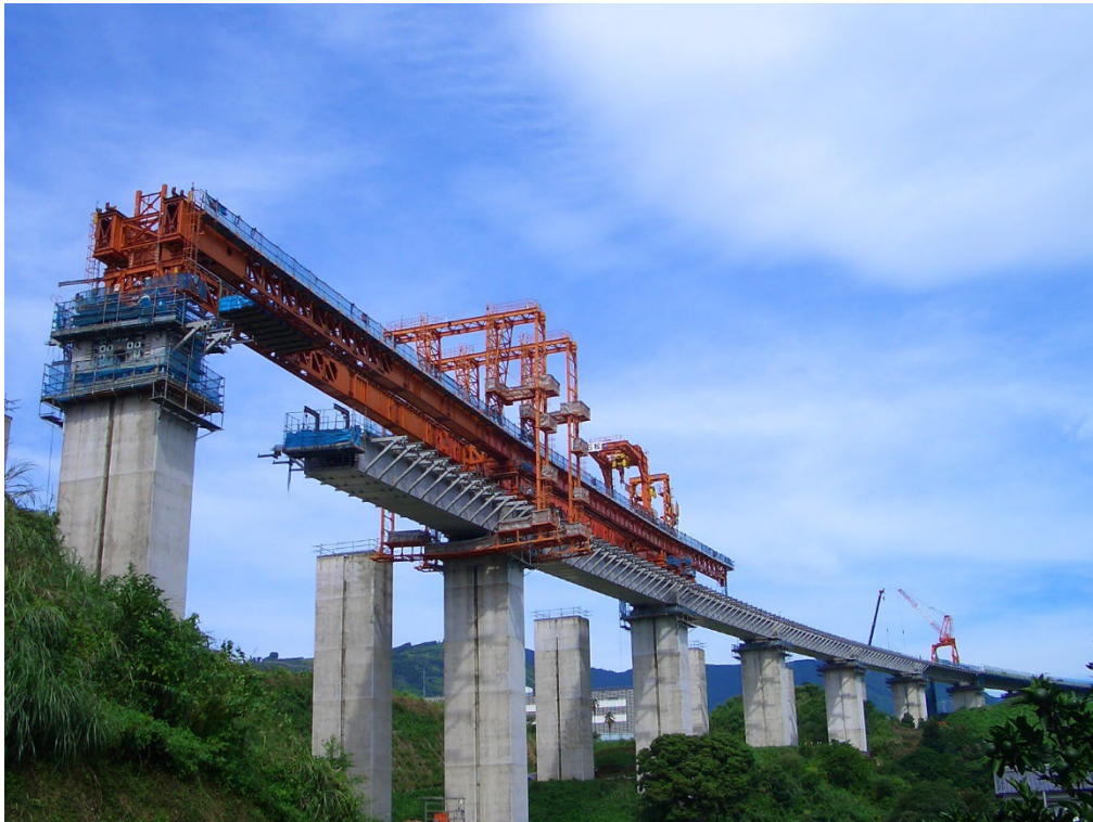
Figure 18 Precast segment cantilevering with erection girder
