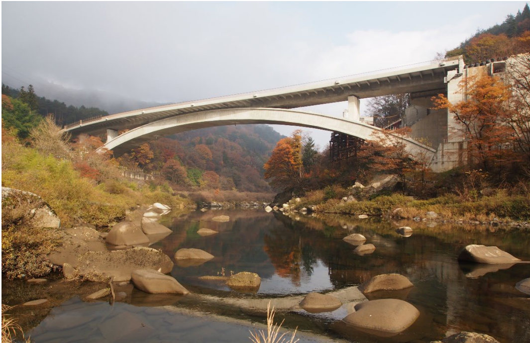
Figure 13 Kakehashi Ichigou Bridge with concrete arch
