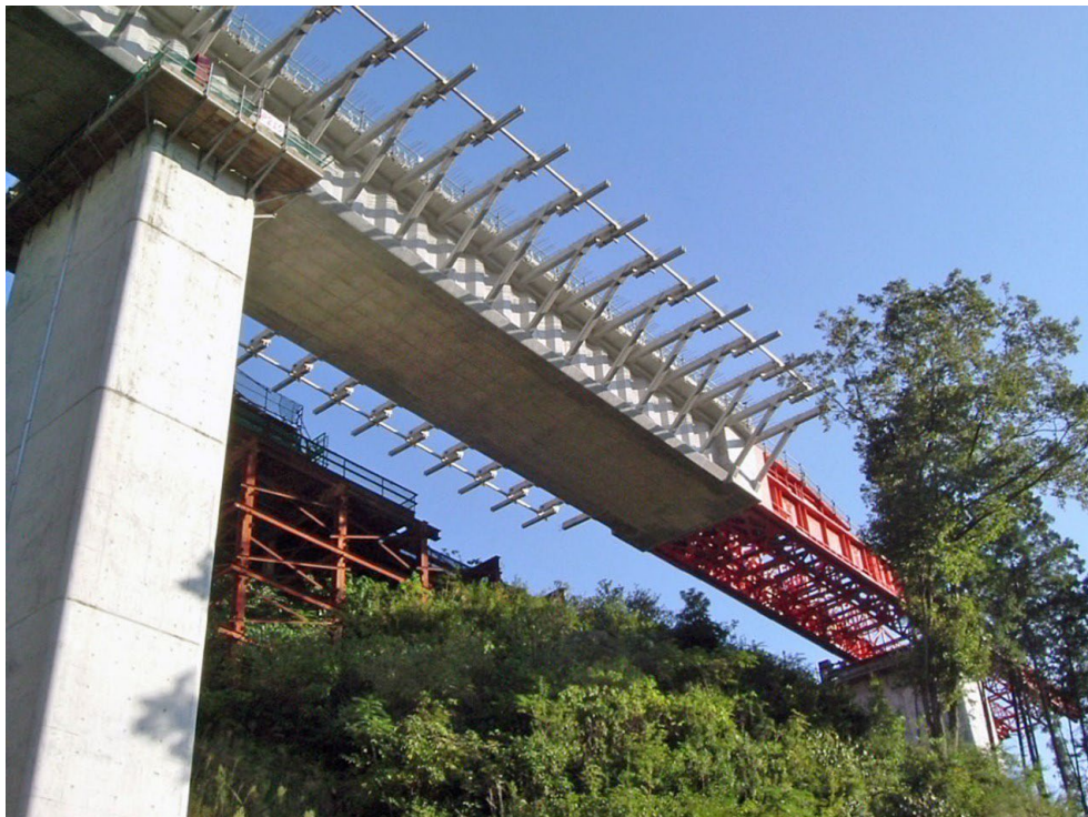
Figure 11 Katsurajima Viaduct by incremental launching of core segments
