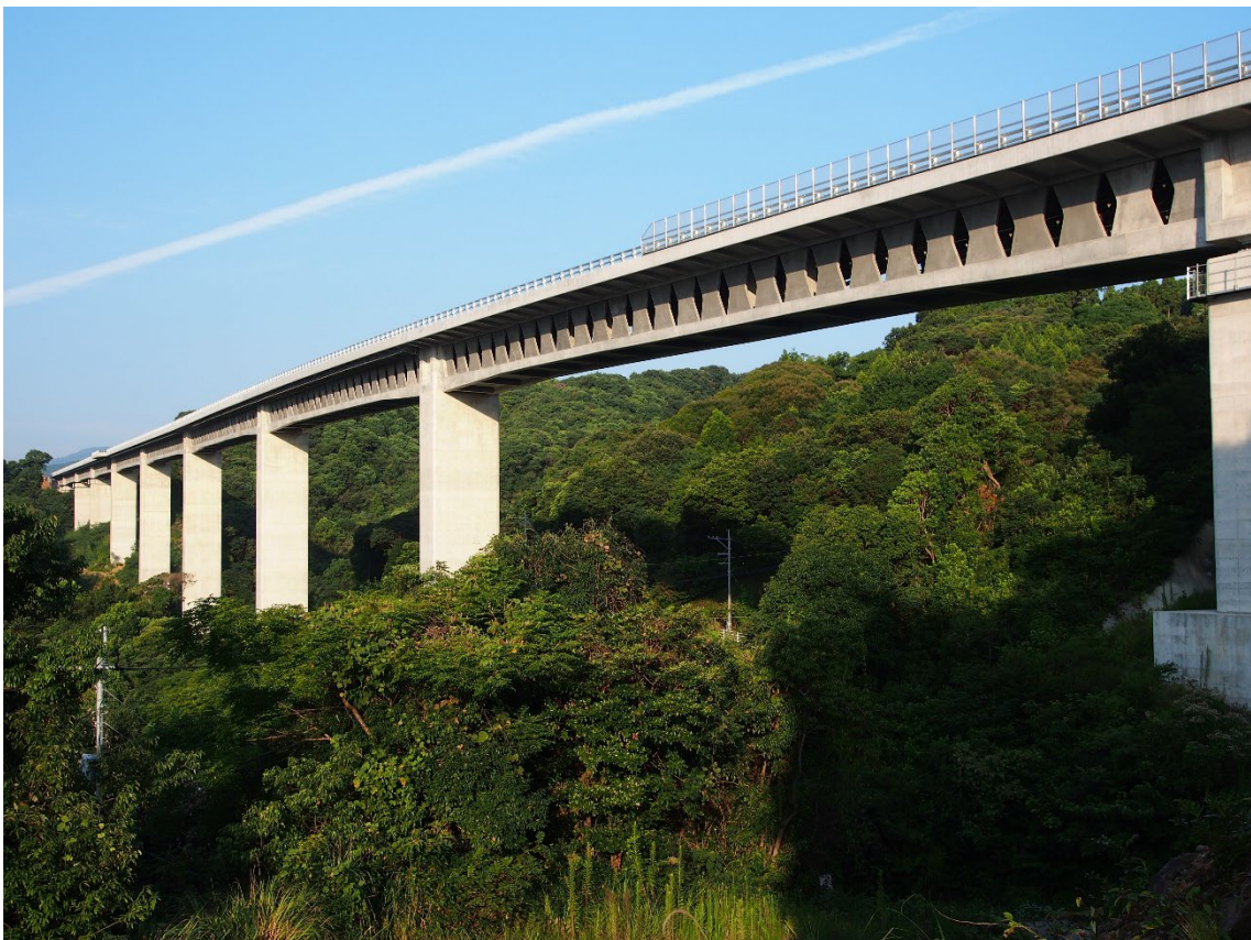
Figure 16 Takubogawa Bridge with butterfly web
