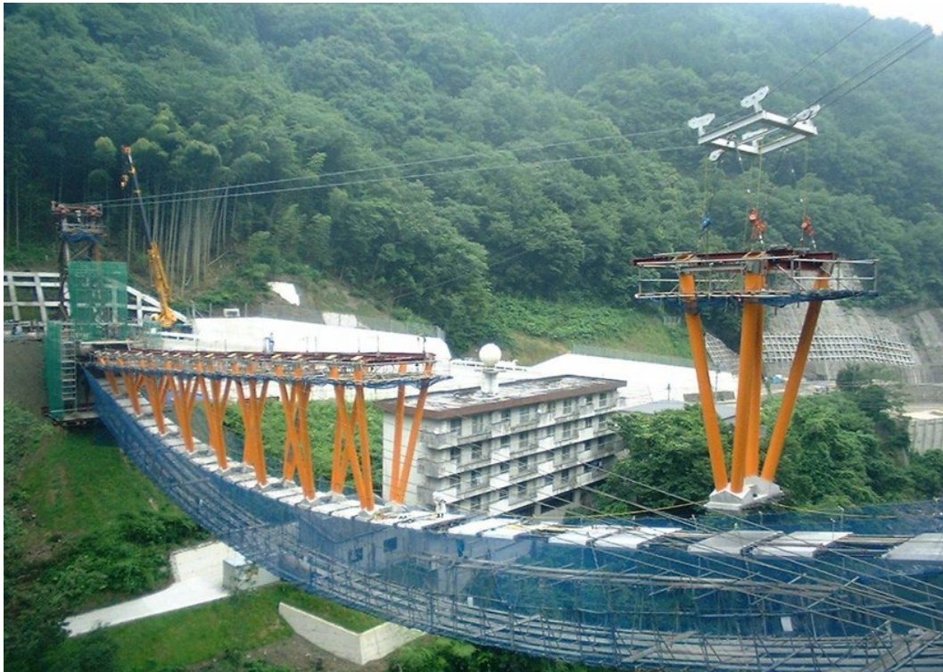
Figure 6 Installation of precast member using suspension cables
