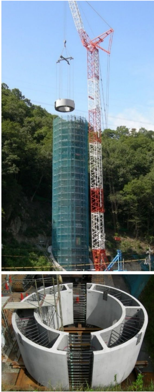
Figure 23 Half precast erection of 80m high pier
