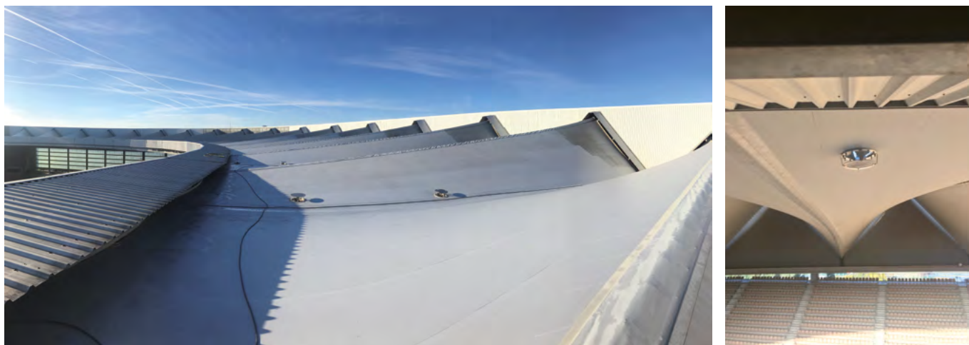
Figure 8. Drainages holes. Credit: schlaich bergemann partner.
