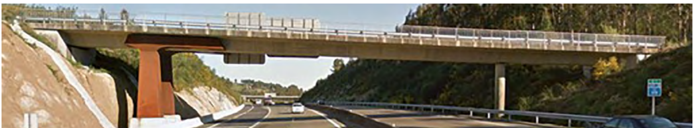
Figure 14. Asymmetric span enlargement in the AP-9 (Pontevedra).
