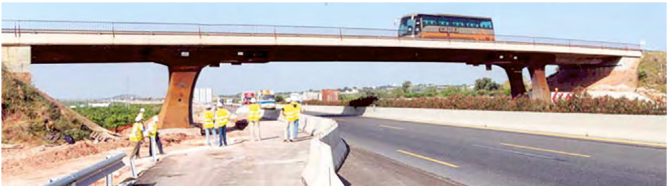
Figure 12. General view of a structure on the A-7 highway in the Valencia By-Pass.
