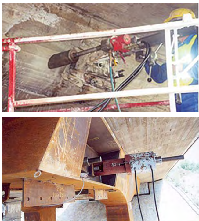
Figure 7. Drilling of deck (top) and tensioning of prestressing bars (bottom).
