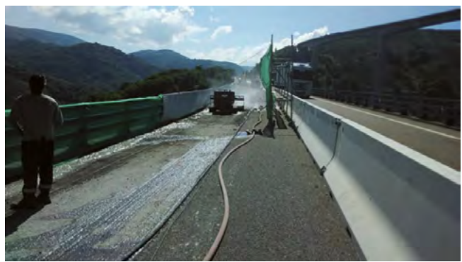
Figure 19. Partial hydrodemolition of the deck.
