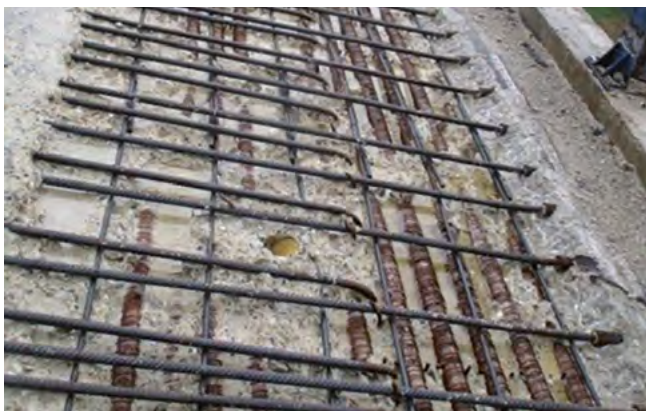
Figure 24. Existing and exposed post-tensioned sheaths.
