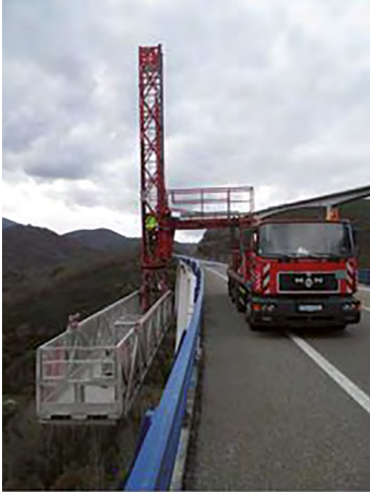
Figure 3. Walkway used in detail inspection.
