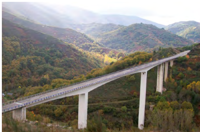
Figure 1. General view once the parapet has been replaced.
