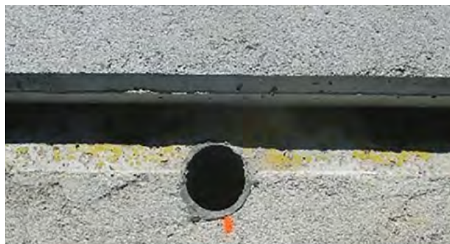
Figure 38. View of newly installed parapet.
