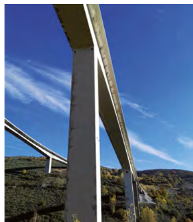
Figure 46. Bottom view of rebuilt deck.
