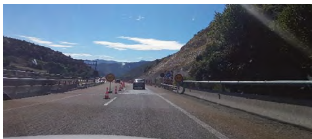
Figure 45. View from Madrid Side Abutment.
