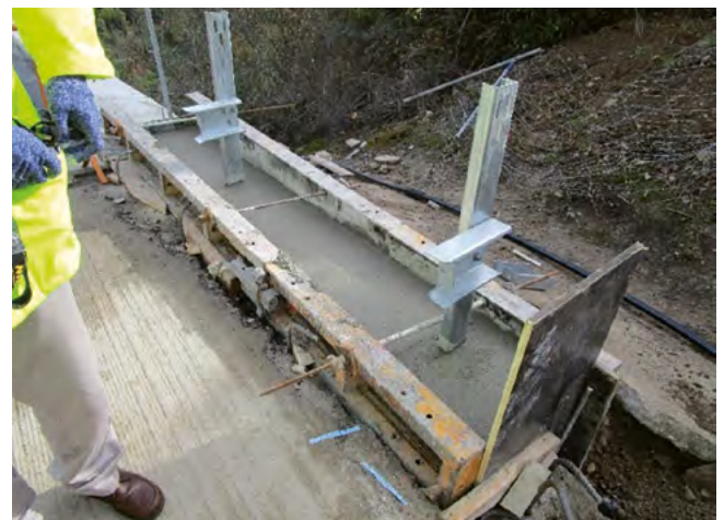
Figure 43. Concrete straps in the abutment area.
