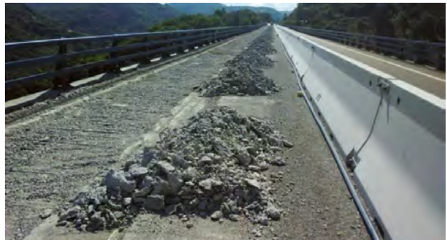
Figure 21. Cleaning hydrodemolition deck residues.
