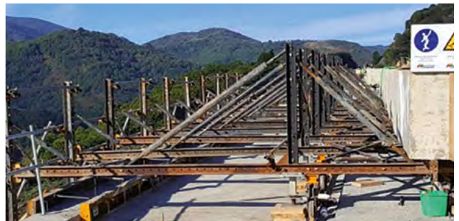
Figure 32. View of the formwork traveler.
