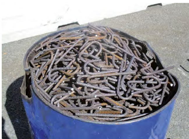
Figure 36. Storage of hooks for fixing bars.
