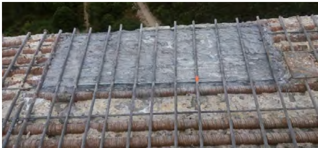
Figure 27. Sealing of deteriorated sheath areas.
