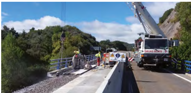
Figure 29. Removal of cut "modules".
