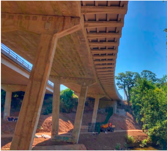
Figure 4. Bromley Heath Viaduct's widening.
