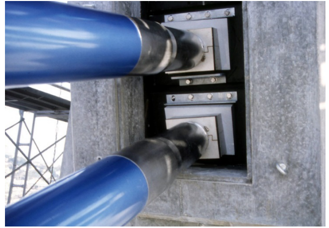
Figure 2. Saddle anchorage of extradosed cables
