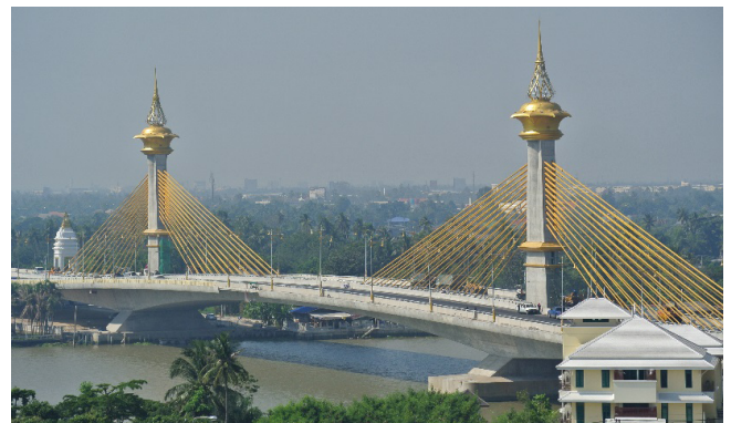
Figure 15. Nonthaburi Bridge (Thailand)
