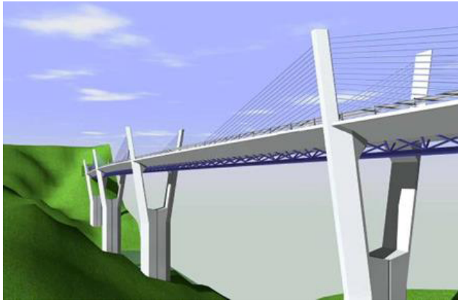
Figure 22. Hybrid combining concrete and space truss
